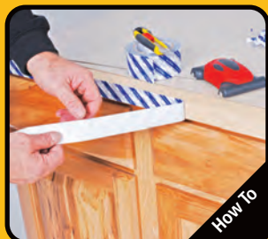
Remove liner, apply edgebanding
