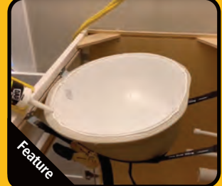
Ratchets hold sink for install prep
